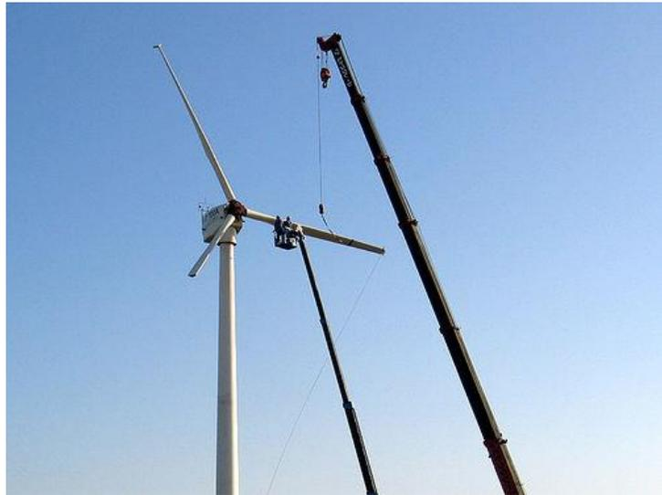
The cost for replacing a gearbox in a 660 kW turbine, on a 65 meter tower, is on the order of \$120,000, for a site with local hydraulic crane service. The bulk of this cost, perhaps 80%, is for procuring and overseas shipping the new gearbox, and the remainder is for crane, site labor and local shipping. Overhauling the gearbox at a local rebuild shop can reduce the total replacement cost to around \$40,000 - \$50,000; these facilities are
